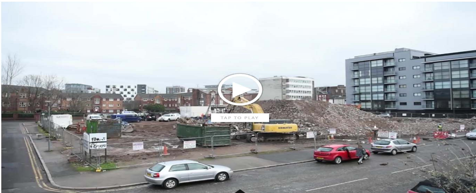
PALL MALL DEMOLITION WORK
